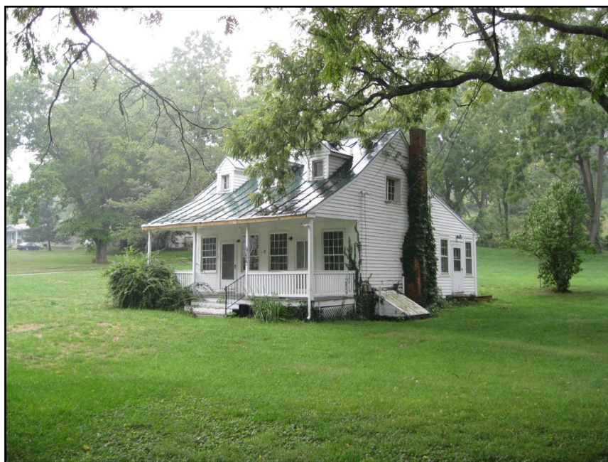
The home of Joseph Funk in Singers Glen, VA was erected about 1810. It was constructed of logs and sheathed with weatherboard. In November of 1974, the home was placed on the National Register of Historic Places. (Photo by SAM 2010)
